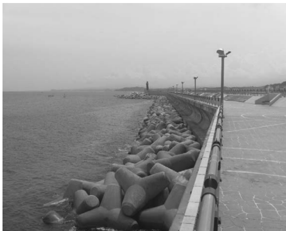
Fig. 8. Application case about recurved wall
