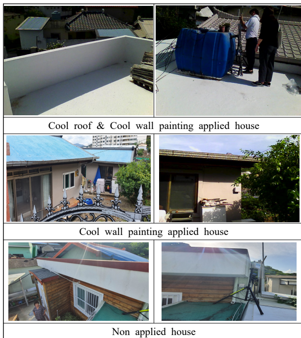
Fig. 6. Installation of external data logger equipment in combined application, cool wall application, and non-applied household
