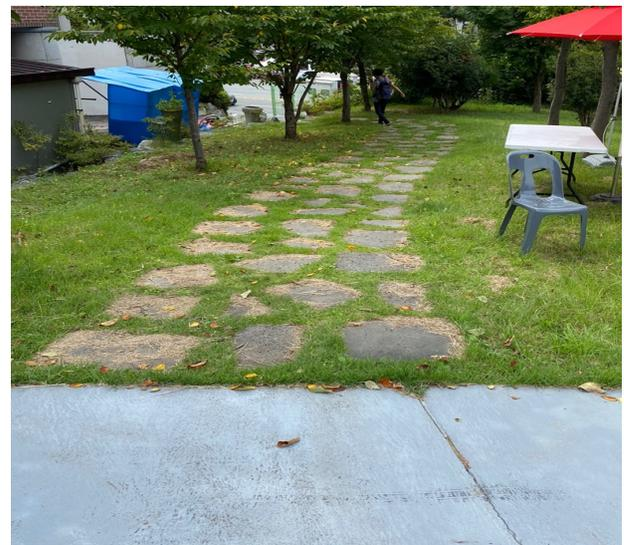
Fig. 1. Cool pavement (down) & Grass block (up)
